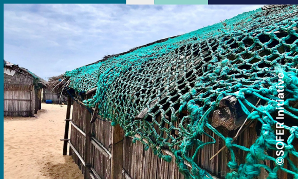
Figure 17: A repurposed fishing net being used to protect a thatched roof in a village in Nigeria.
