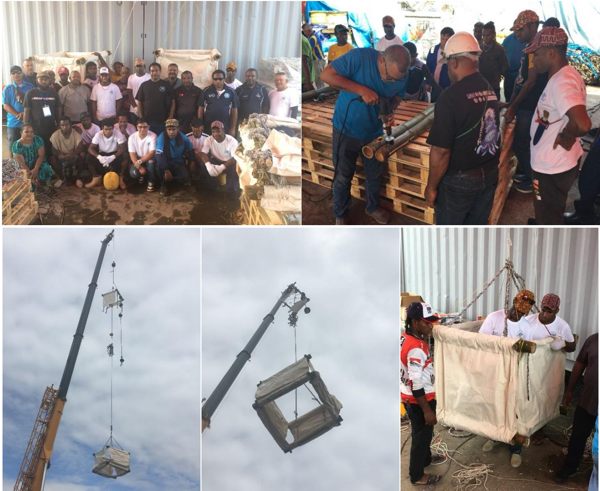
Figure 12. Jelly-FAD construction workshop in Lae, at Frabelle fishing companies compound in Lea (PNG) in July 2024.
