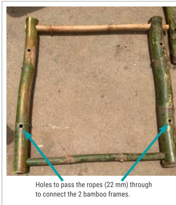
Holes to pass the ropes (22 mm) through to connect the 2 bamboo frames.
